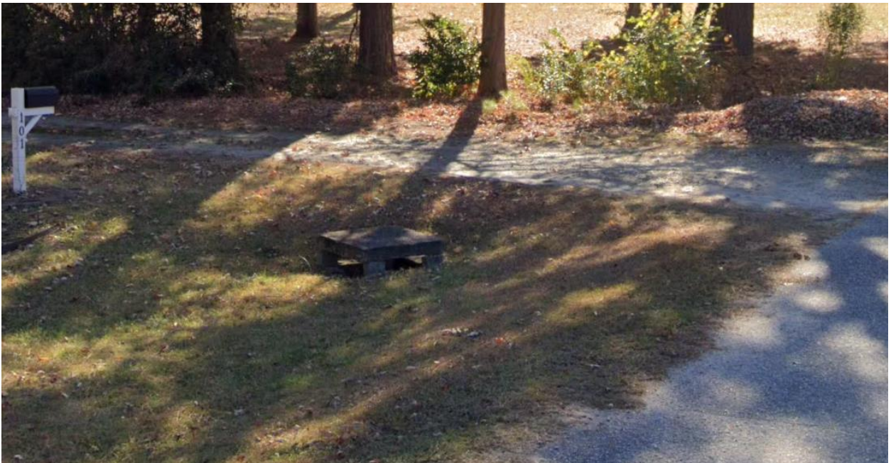
Existing yard inlet to be modified to receive the re-graded ditch line.
